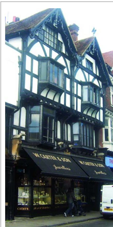
Fig 20: A traditional retractable blind that reflects the character of the shop and does not detract from the upper stories of the building. Because the fascia is covered when it is open, the business name is printed on the blind.
