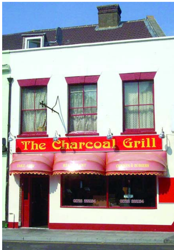
Fig 19: A modern Dutch canopy in plastic and a fascia in garish colours. The fascia sits uncomfortably close to the first floor windows with a bank of visible swan-neck lights. A retractable blind with the business name written on the blind would have been preferable.
